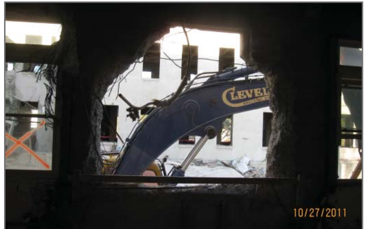
View from inside C, D, and F Wings during interior demolition.
