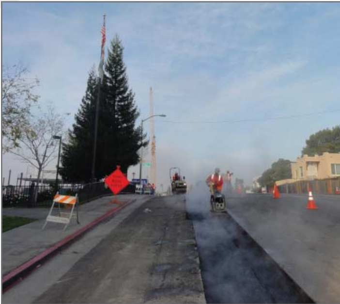
Utility work on East 31st Street.
