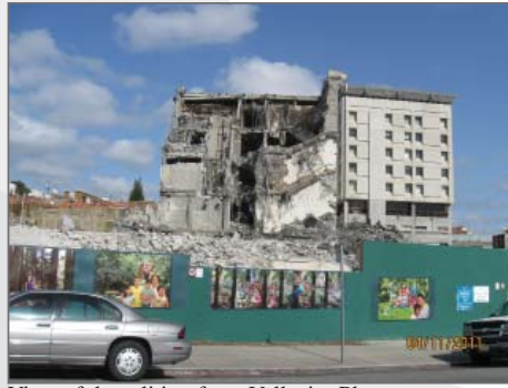
View of demolition from Vallecito Place.
