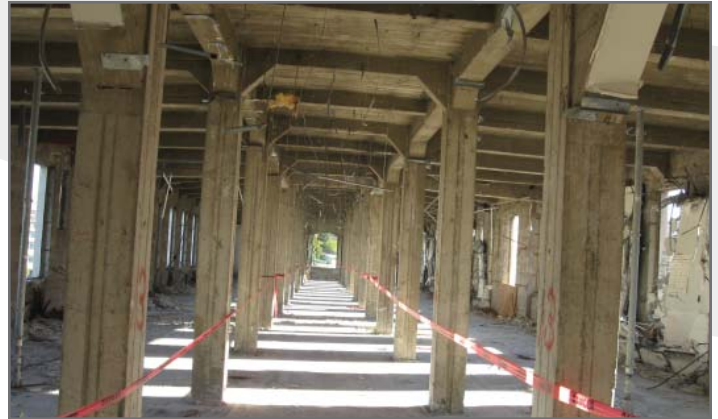
Interior demolition of C, D, and F Wings in progress.
