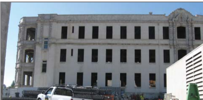
View of exterior shell ready for demolition.
