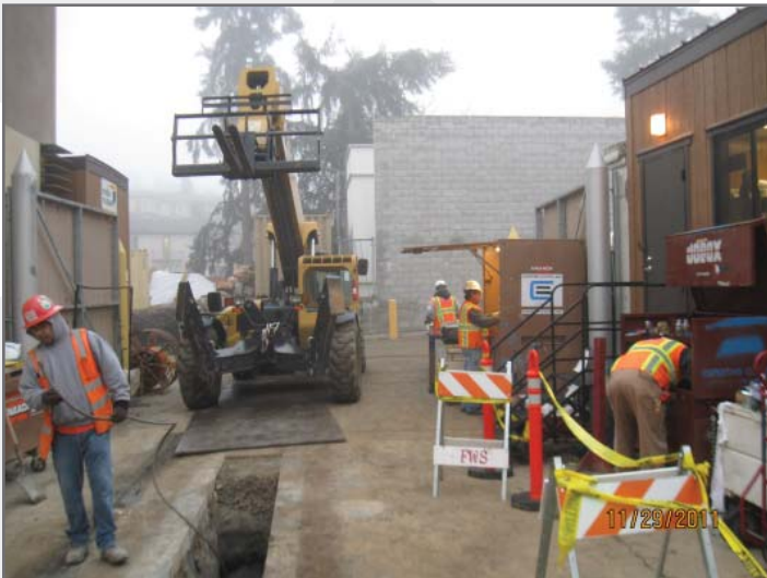
Utility work between C, D, and F Wings.
