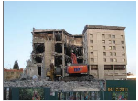
View of demolition from Vallecito Place.
