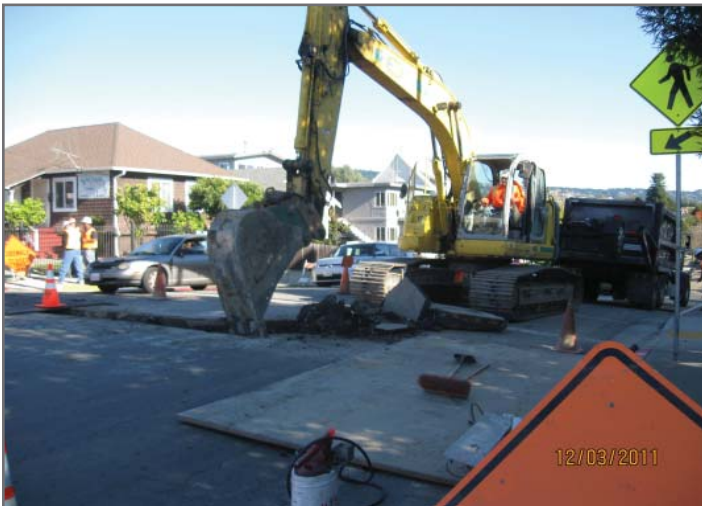
Utility work on East 31st Street and Stuart Street.
