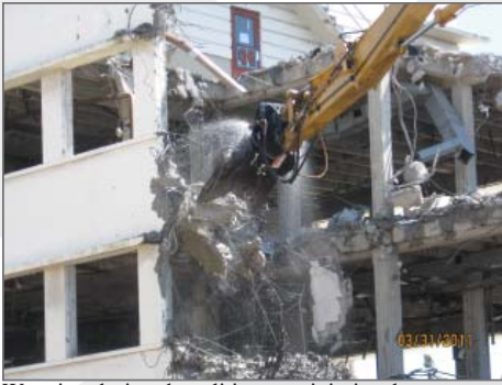
Watering during demolition to minimize dust.
