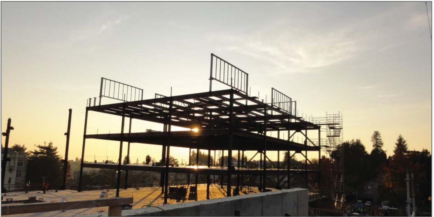
Structural steel in progress.
