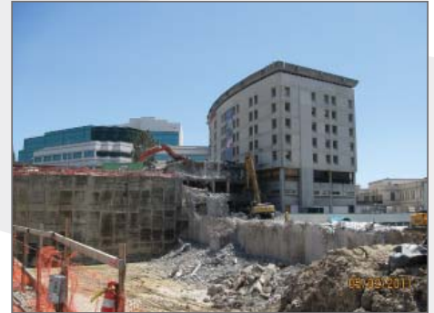
After completion of V Building demolition.
