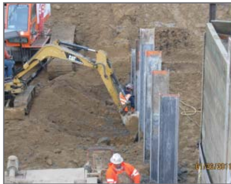
Placing steel beams into the holes.
