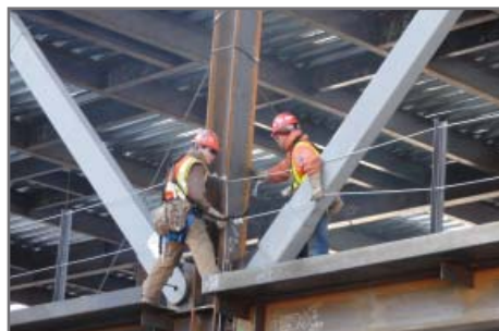
Steel contractors using proper safety gear.
