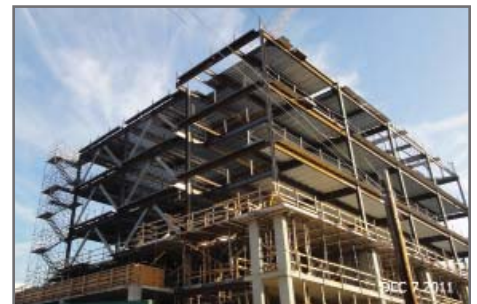
Structural steel in progress.
