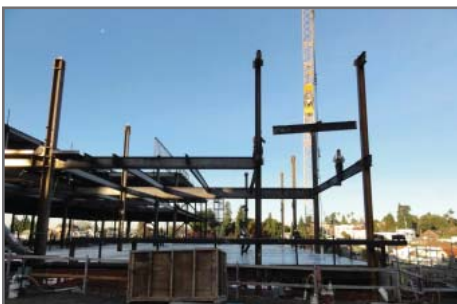
Placing structural steel beam
