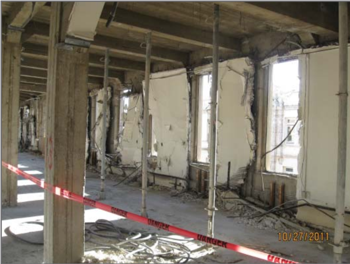
Interior demolition of C, D, and F Wings in progress.
