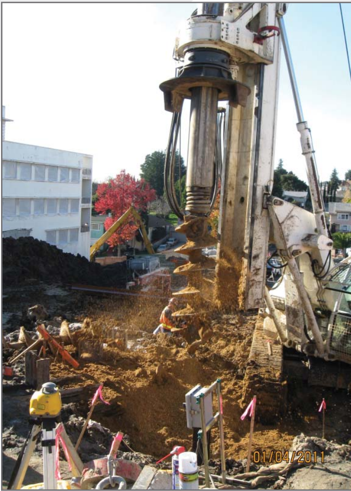
Drilling into the ground to start shoring.
