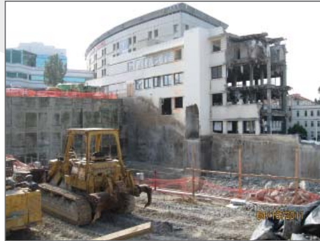
View of demolition from inside construction fence.
