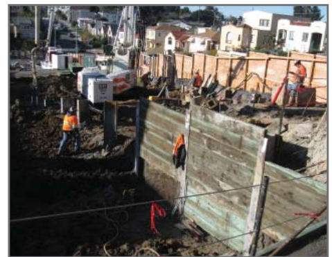
Pushing the beams down to foundation level.
