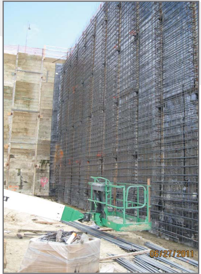
The shoring at final stage.
