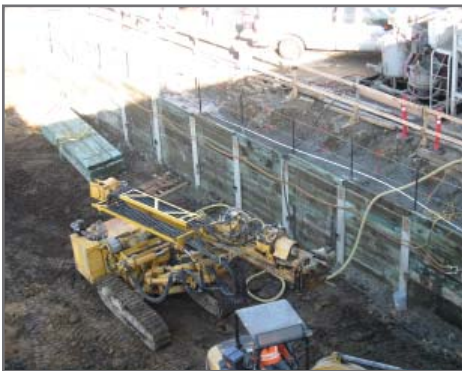
Placing wood planks between the steel beams.
