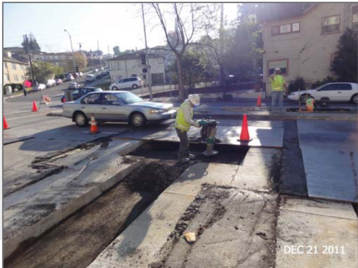
Utility work on 14th Avenue.
