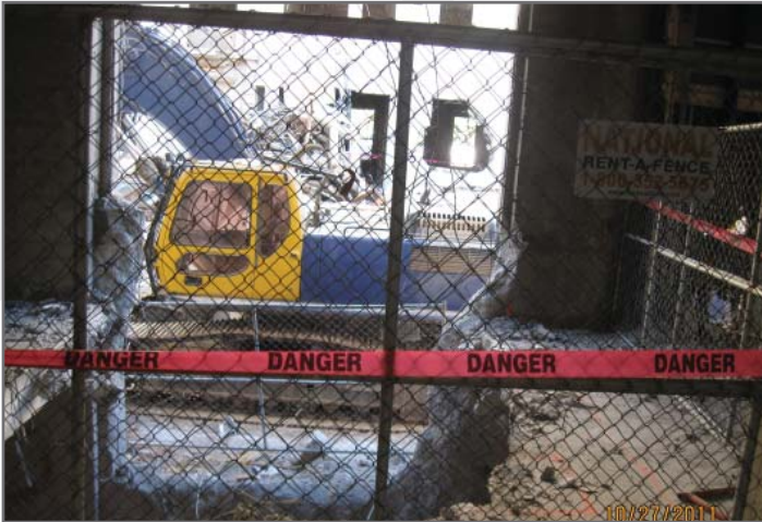
View from inside C, D, and F Wings during interior demoli-
