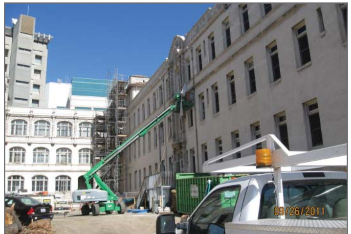
Removal of terra cotta for reuse.
