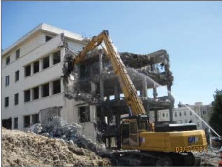
Watering during demolition to minimize dust.
